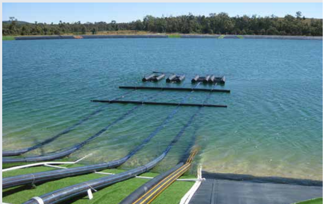
CSG industry dam showing engineered layers.
