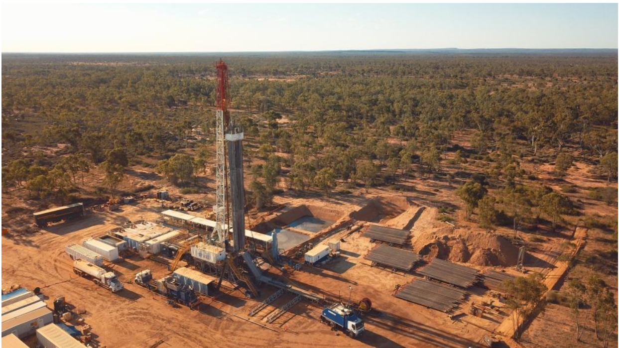
Figure 1 – Ensign Rig 932 on site at Albany 2
