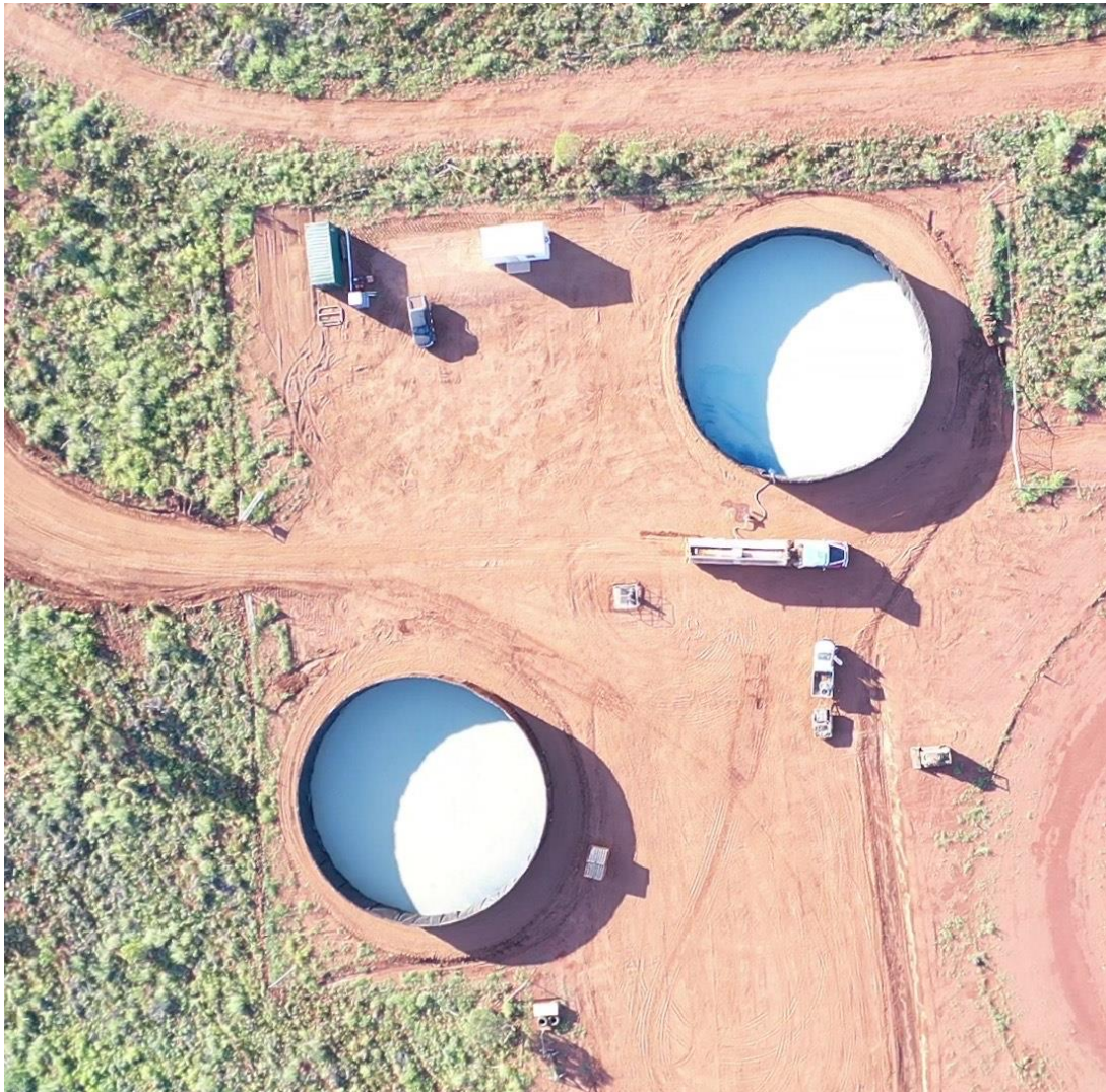
Figure 1: aerial shot of the installed water tanks with the Mahalo North 1 wellhead in the central area between the tanks
